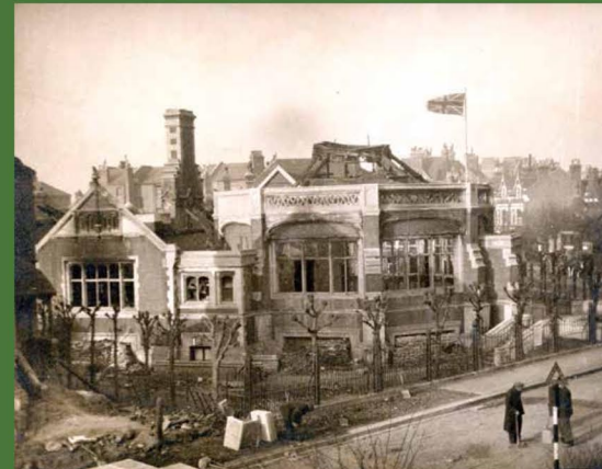
Bomb damage at the Minet Library
